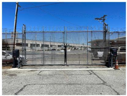
1. Locate the reset/disconnect switch on both sides of the gates.
